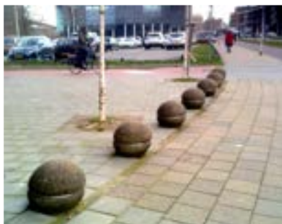
4.7.2. grooved concrete spheres preventing undesired parking of cars in the premises of the Leiden University Teaching Hospital, the Netherlands, 2020 CE
